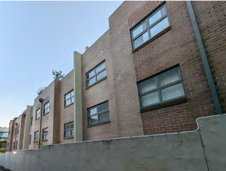
Rear of 15-41 Cornwallis Street
