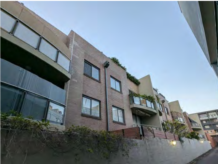
Rear of 15-41 Cornwallis Street
